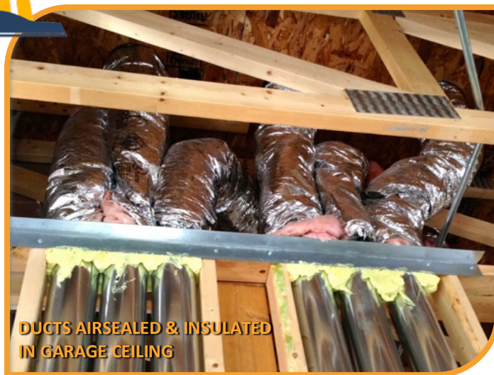
GARAGE PROVEN DISCONNECTED WITH ZONAL PRESSURE TEST
