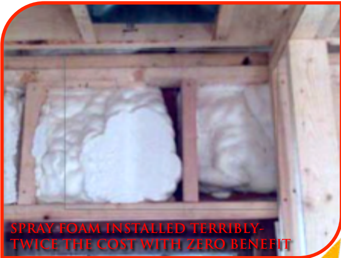
NO AIRSEAL AT PORCH CONNECTION
