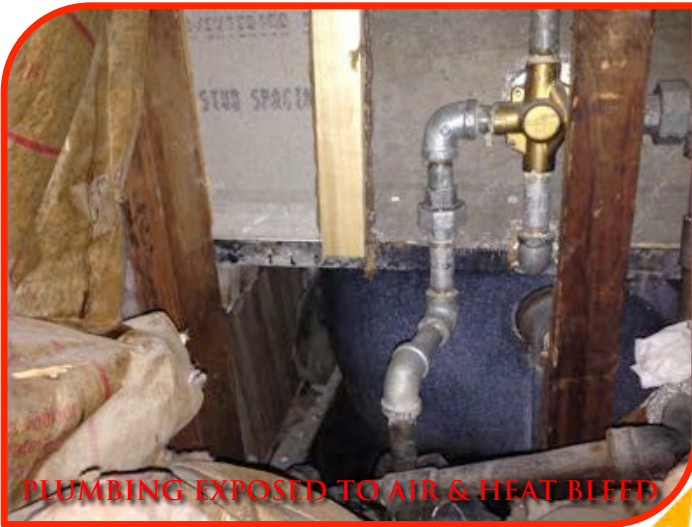
MISSING AIR BLOCK IN FLOOR CAVITY
