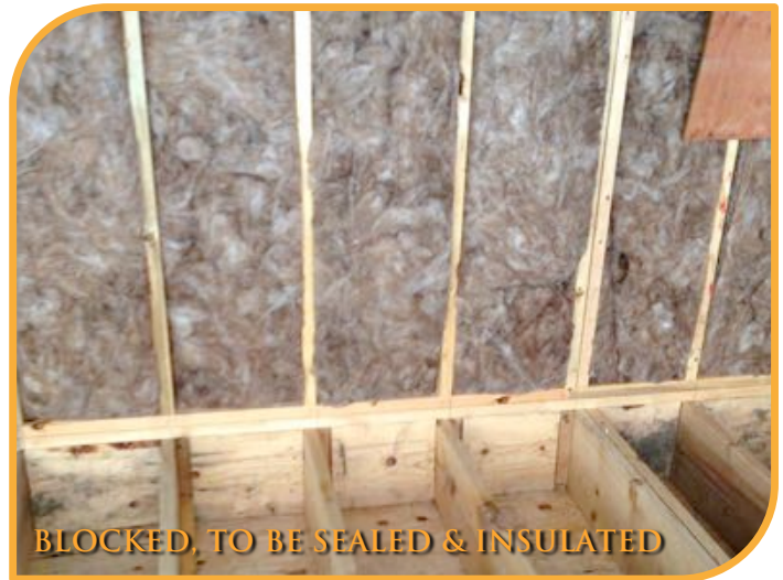
MISSING AIR BLOCK IN FLOOR CAVITY
