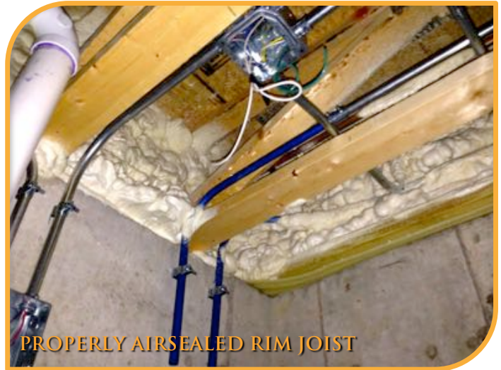
RIM JOIST FRAMING VERY DIFFICULT TO AIRSEAL
