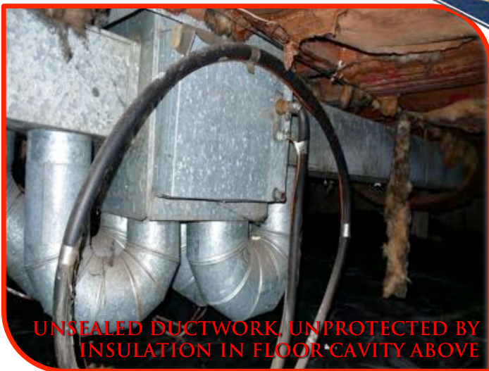
INSULATED AGAINST THE HOME (CEILING) AND AGAINST OUTDOORS (WALL) PICK ONLY ONE - INSIDE OR OUT!
