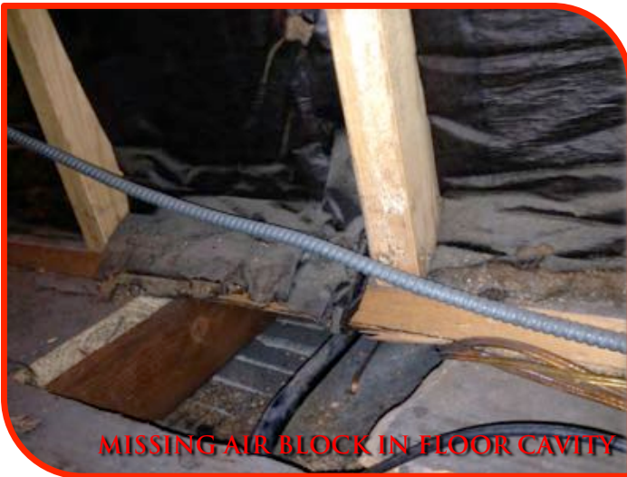
BLOCKED, TO BE SEALED & INSULATED
